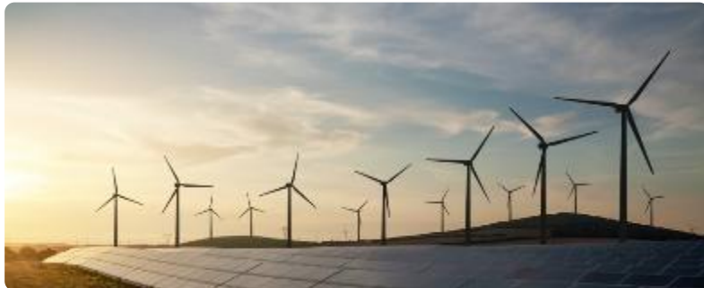
Renewables & Energy Storage (Wind, Solar, BESS)
