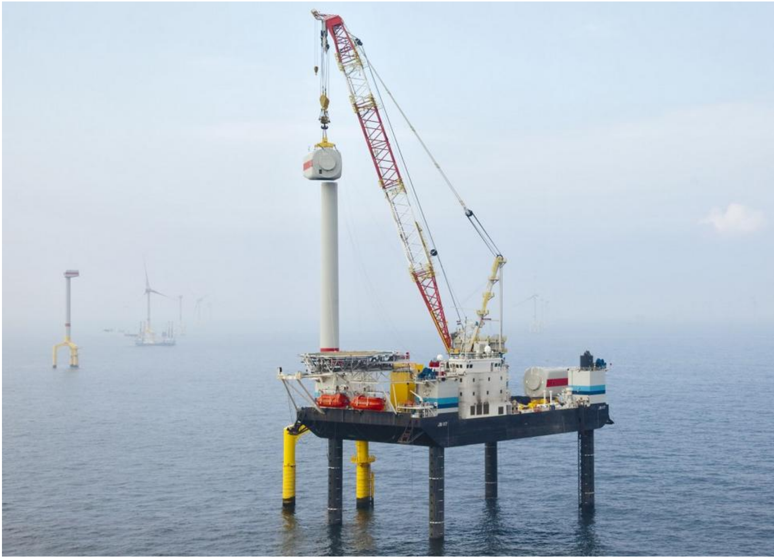
Jack-up vessel for wind park installation
